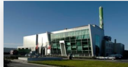
2008 – 3 MW el ORC turbo-generator for heat recovery on a waste incinerator in Belgium
