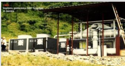
1988 – 200 kW el ORC geothermal plant in Zambia
