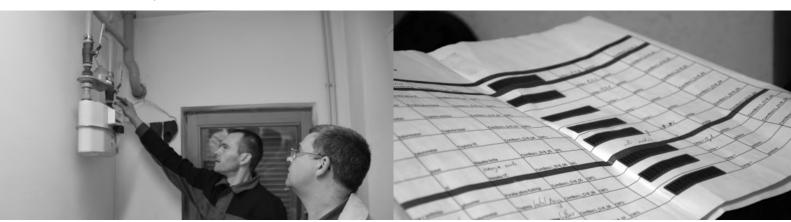
Combox.L communication devices collect data from meters in regular 15-minute intervals and transmit the readings via the "LoRa" network to gateways, which then transmit them to the EMS (Energy management system). This is all done using the standard LoRaWAN communication protocol.
