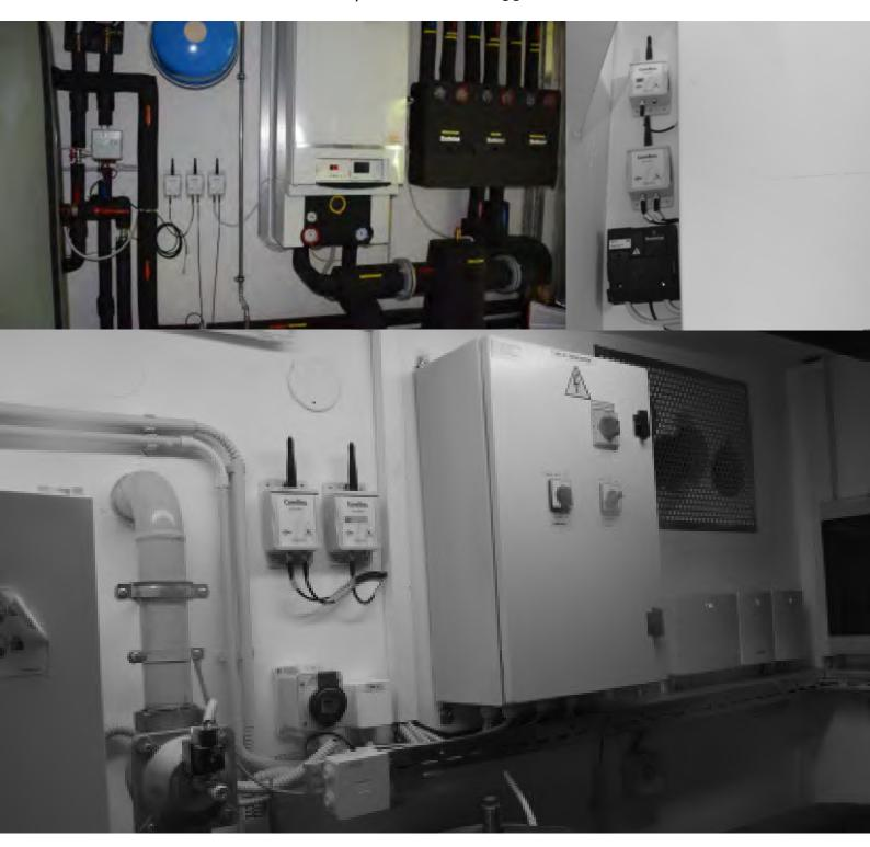
During the energy renovation process of the complex, they ordered an energy use monitoring and management system. The distances between individual meters and the position of the building made wired communication unsuitable. We used the wireless ComBox.L communication devices to set up communication with the energy management system.
