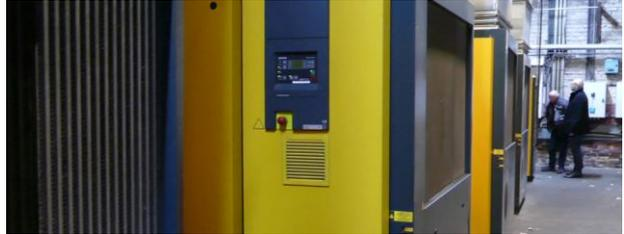
Second, let's look at an industrial signage production facility where we installed a 1.2 MW compressed air system. Heat recovery uses heat exchangers installed on the tops of the compressors. This configuration was preferred to take advantage of the available space. The total recovered energy is around 800 kW for the complete system. It is reused in the customer's heating system."
