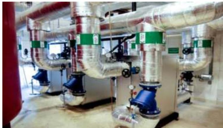
SWEP's ETS: 3x6MW units connected in parallel.
