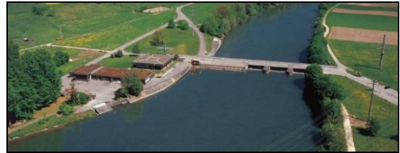
Figure 1: Bannwil Hydropower Station (Source: Onyx Energie Mittelland)
