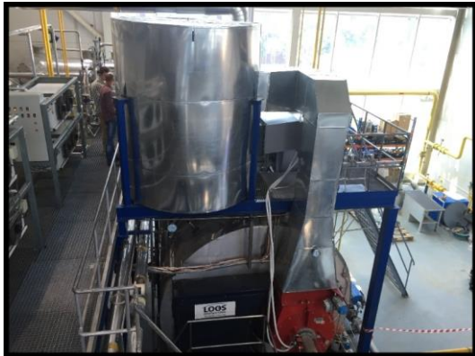
The HeatMatrix polymer LUVO heat exchanger installed on the LOOS steam boiler at Carlsberg, Kiev.
