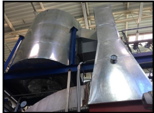
The HeatMatrix polymer LUVO heat exchanger installed on the LOOS steam boiler at Carlsberg, Kiev.
