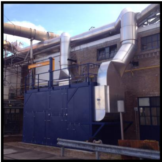
The skid in operation. The design of the skid with 3 heat exchangers.
