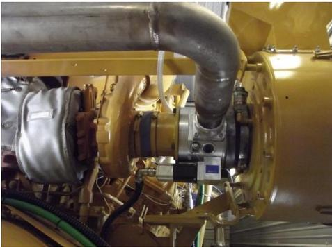
*Caterpillar G3516B equipped with VariFuel2 air/fuel ratio mixer*
