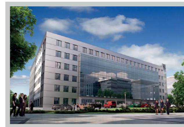
West House 1 B, Archicom
